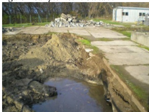
Figure 1 Sample No. 2. Oil tank
