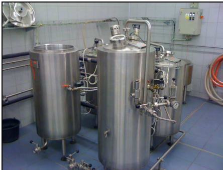
Figure 1: Fermentation part of Destila micro-brewery assembly. Note the cylindroconical fermenter in the foreground with extensive piping accessory (position of SENSOR2). Photo by D. Varner
